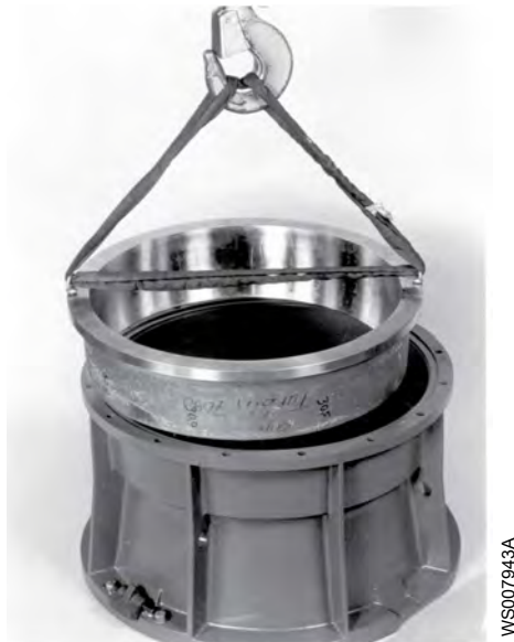
Figure 22: Lowering the wear ring into the outlet cone
